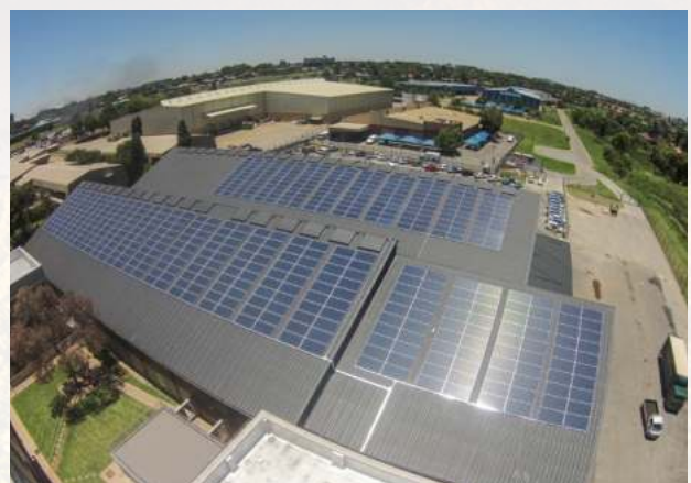
Solar panels on the roof of the warehouse in Johannesburg.
